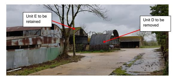
'Existing Unit E (proposed Unit D) is a steel framed shed, rectangular on plan and open on 3 sides. It is linked to the adjacent Unit D on the East side by a monopitch roof which will not be retained in the proposed development. Unit E (proposed Unit D) measures approximately 23m x 9m and is 4.5m to eaves. The roof is pitched and gabled with a central ridge running north/south and steel trusses supported at each end on posts.'
